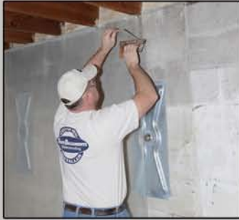
1. Preparing wall (attaching a vapor barrier)
