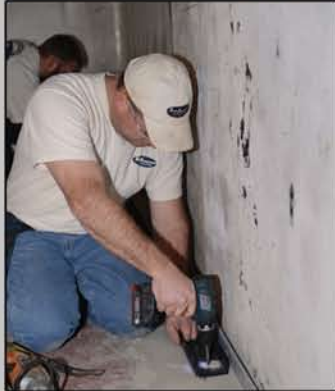
3. Attaching E3 Wall Base channel
