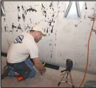
2. Laying out E3 wall for installation
